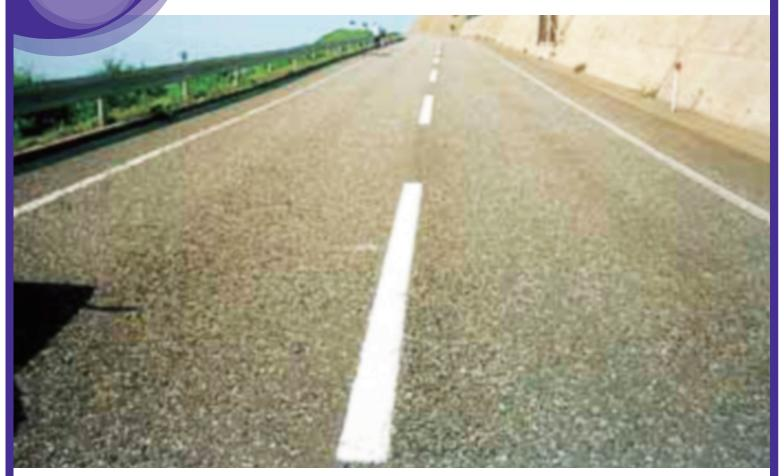
This is a pavement where single-sized aggregate is dispersed and pressed-fitted in a dense mixture. A mixture type is also available.
